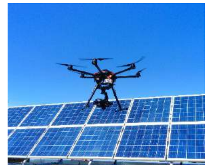
Figure 1- Drone equipped with an InGaAs camera for EL inspections
